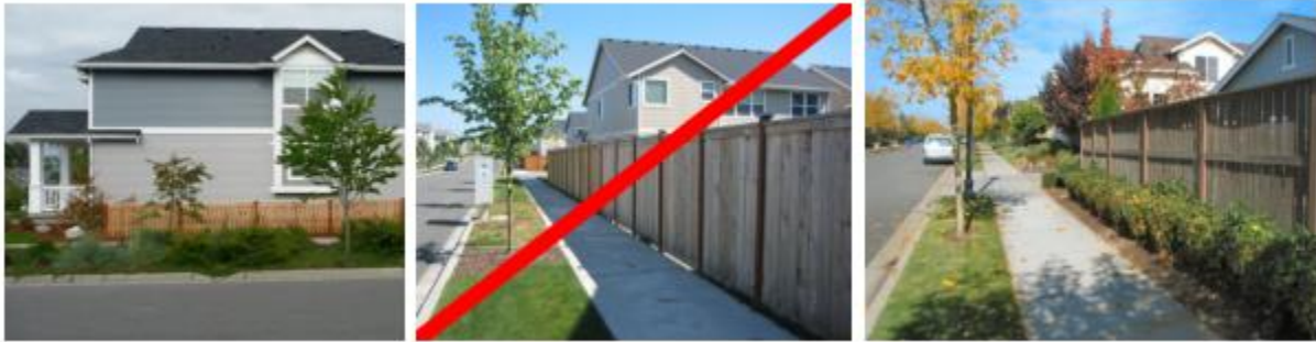
Figure 15.320.130(A)(2). Acceptable and unacceptable fences on corner lots for side yard/flanking streets or along reverse frontage lots where the back yard abuts a street. The left example is a low picket fence. Taller fences like that in the middle image are acceptable along the side and rear yard, but are not allowed within five feet of a sidewalk. The right image shows an acceptable example where the fence is set back away from the sidewalk to allow space for landscaping.
