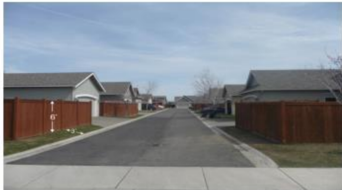
Figure 15.320.130(A)(3). Acceptable fences along an alley. The 42-inch fence on the left is allowed along the edge of an alley. The taller six-foot fence in the middle is allowed with a three-foot minimum setback from the alley.
